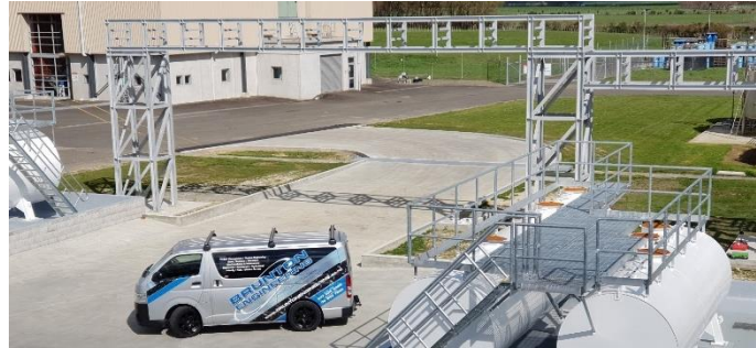
Pipe Bridge fabricated and installed by Brunton Engineering
