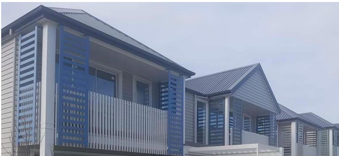
Aluminium louvres fabricated and powder coated by Brunton Engineering.
